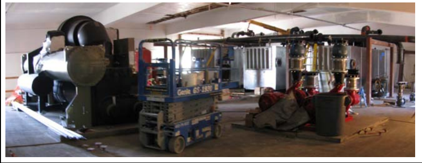
Building 2800 – Central Plant
