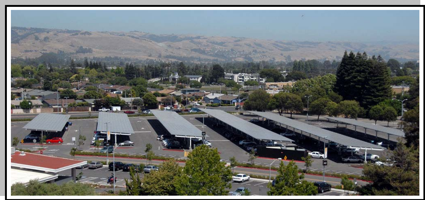
Lot G with Photovoltaic
