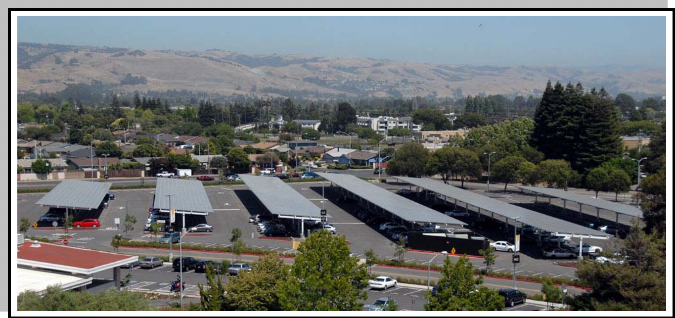
Lot G with Photovoltaic
