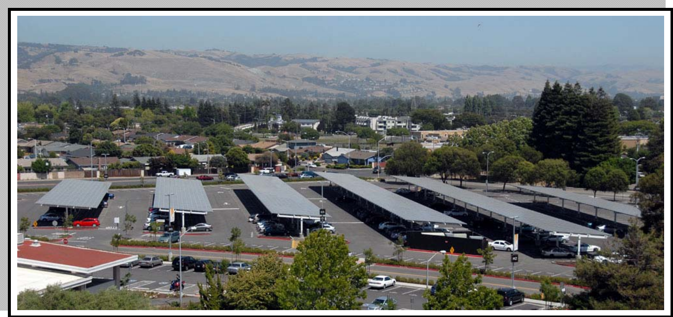
Lot G with Photovoltaic
