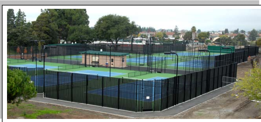
New Tennis Courts
