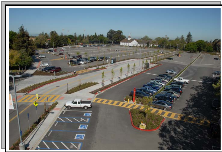
Parking Lots A and B with New Bus Stop.
