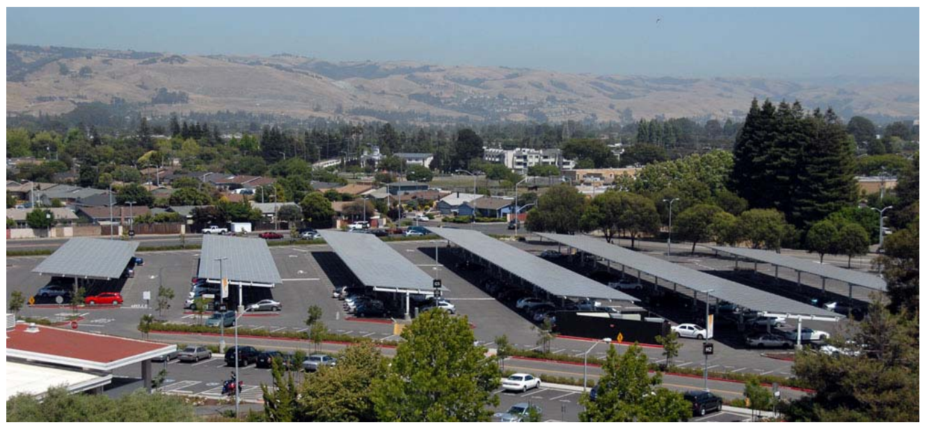
Lot G with Photovoltaic
