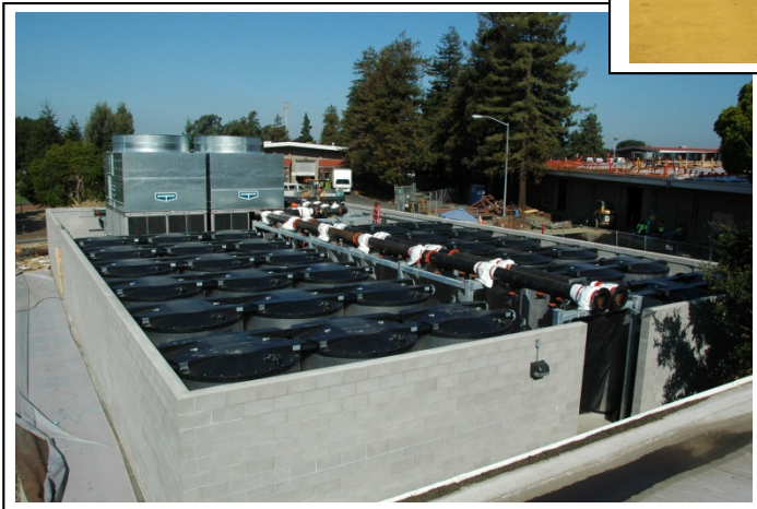
Ice Storage Plant
