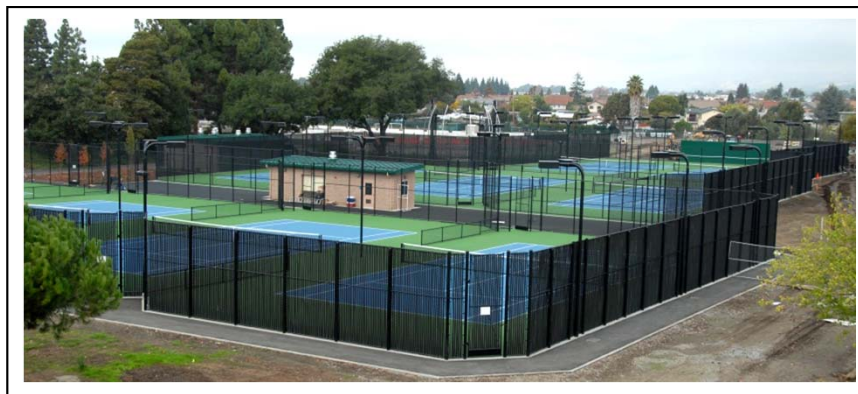
New Tennis Courts
