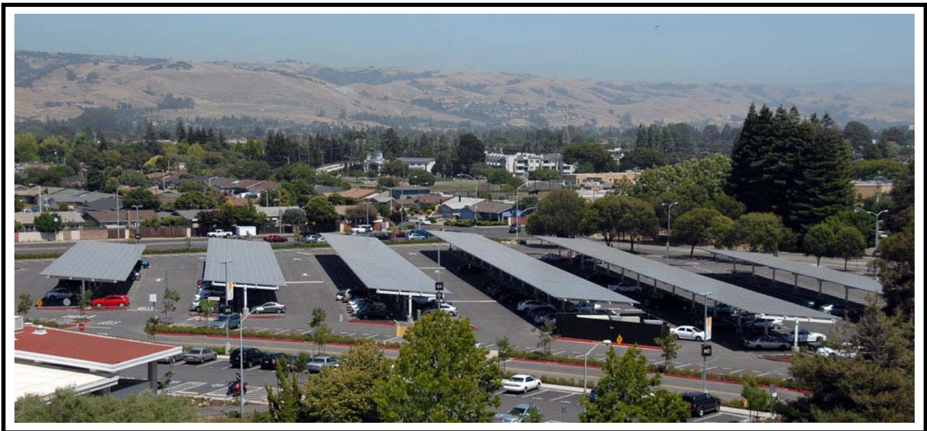
Lot G with Photovoltaic
