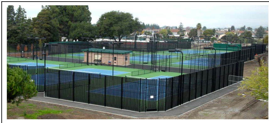
New Tennis Courts
