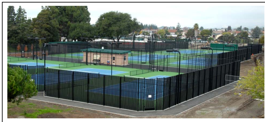
New Tennis Courts
