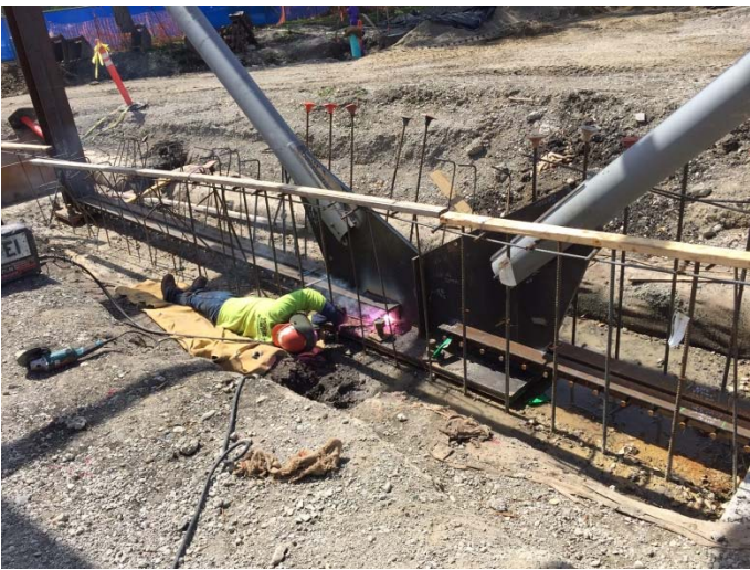
STEEL BRACE FRAME WELDING
