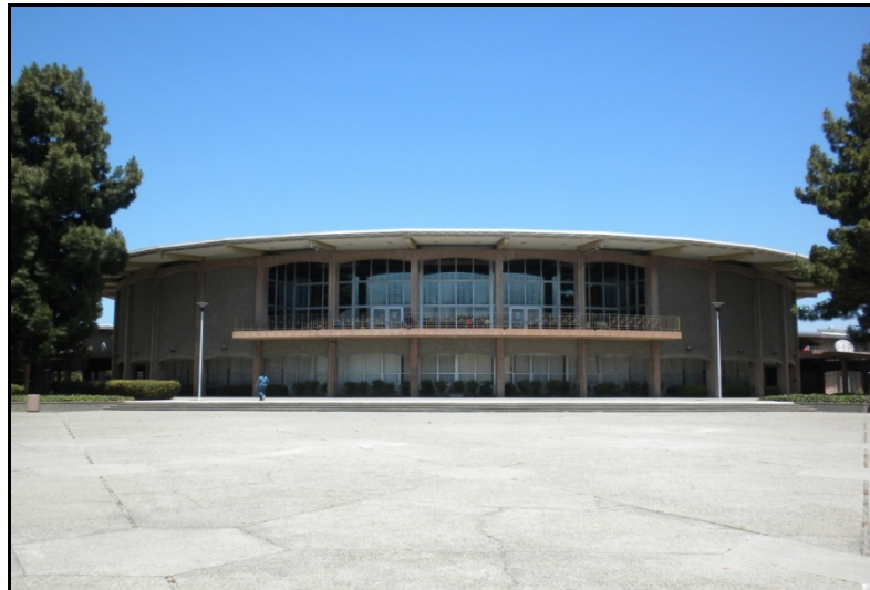
Learning Resource Center Elevator and Library Upgrade
