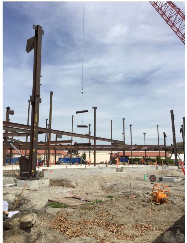
STEEL ERECTION Page 32 of 96
