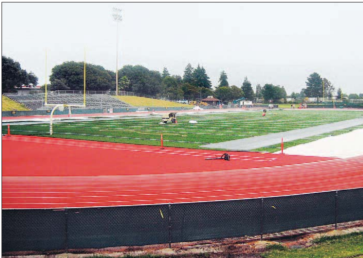
Chabot's renovated football field
