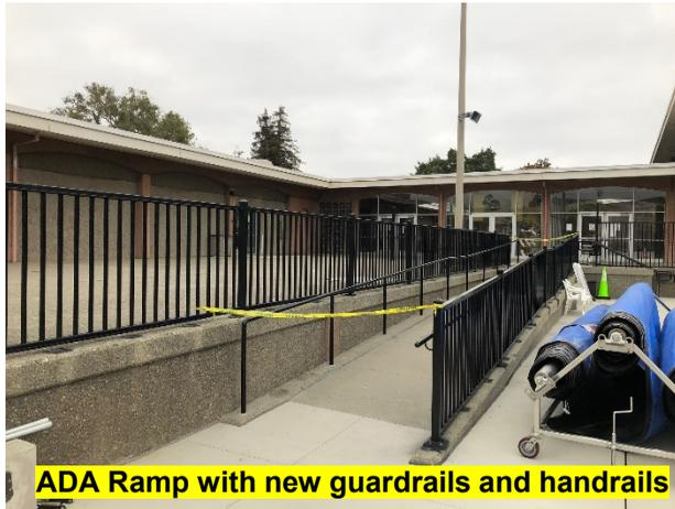
ADA Ramp with new guardrails and handrails
