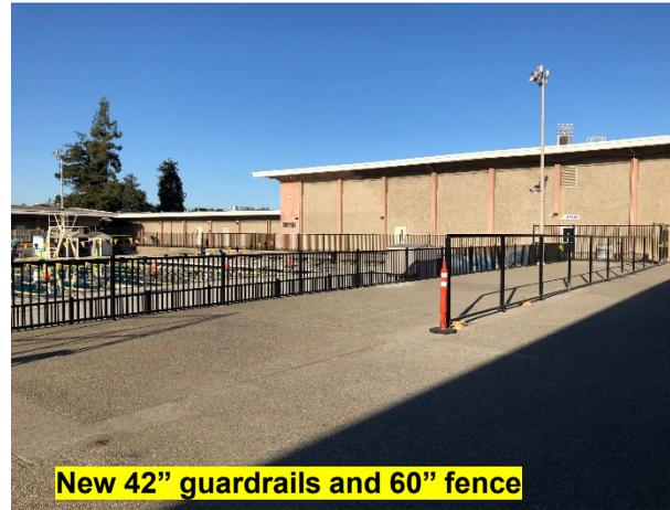
New 42" guardrails and 60" fence
